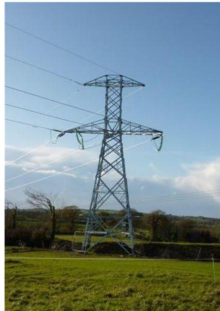
Figure 3.3: Typical steel angle structure
