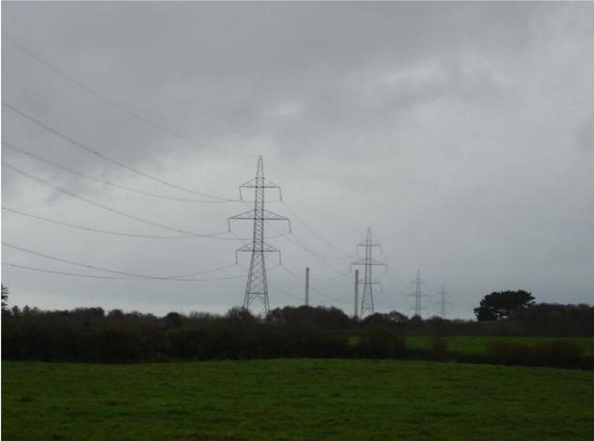
**Figure 3.1: 400kV double circuit intermediate towers near Moneypoint generating station Co. Clare.**
