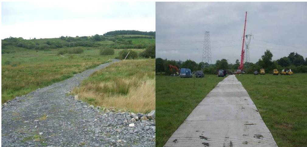
Figure 5.1: Temporary Stone and Aluminium Panel tracks
